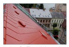
Ventilation of roof frame with plastic ventilation terminals.
