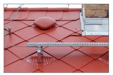
The size in exit hole of plastic cow ventilation apertures is 200 cm<sup>2</sup> /1pc.
