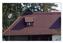
Ventilation of roof frame is by raised roof ridge.
