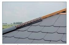
The size of exit hole with ridge ventilation is  $100 \text{ cm}^2$  /m. Air space is 1 cm/m.
