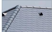
The size of Oriko could ventilation aperture is 100 cm $^2$  /1pc.
